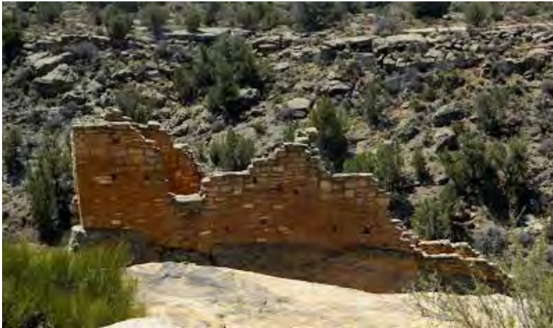
Masonry blocks used to construct the buildings at Hovenweep were quarried from the Dakota Formation – without the aid of steel chisels to shape.
